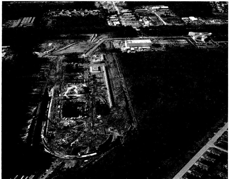
Aerial view showing CEBAF construction progress.
